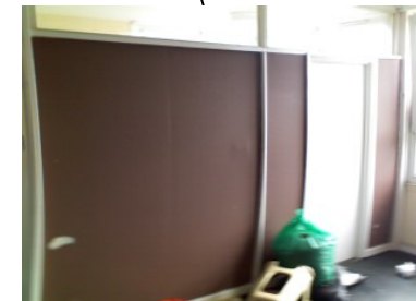
Insulating board as partition wall
