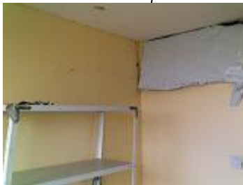
Insulating board as partition wall
