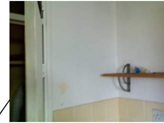
Insulating board as partition wall
